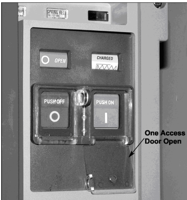
Figure 5-27 Pushbutton Cover Mounted
