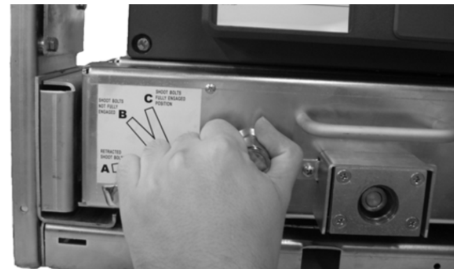
Figure 4-9 Shoot Bolt Handle Shown in Position "A" - Shoot Bolts Retracted Fully Inside Cradle
