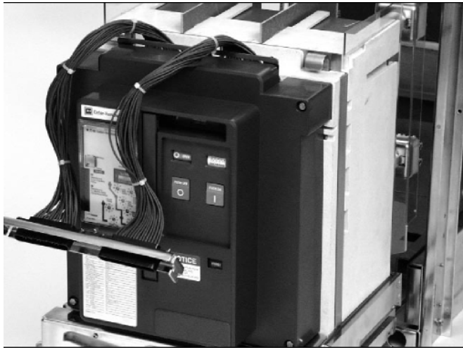
Figure 4-10 Secondary Umbilical Cord Shown Connected to Breaker Prior to Breaker Insertion
